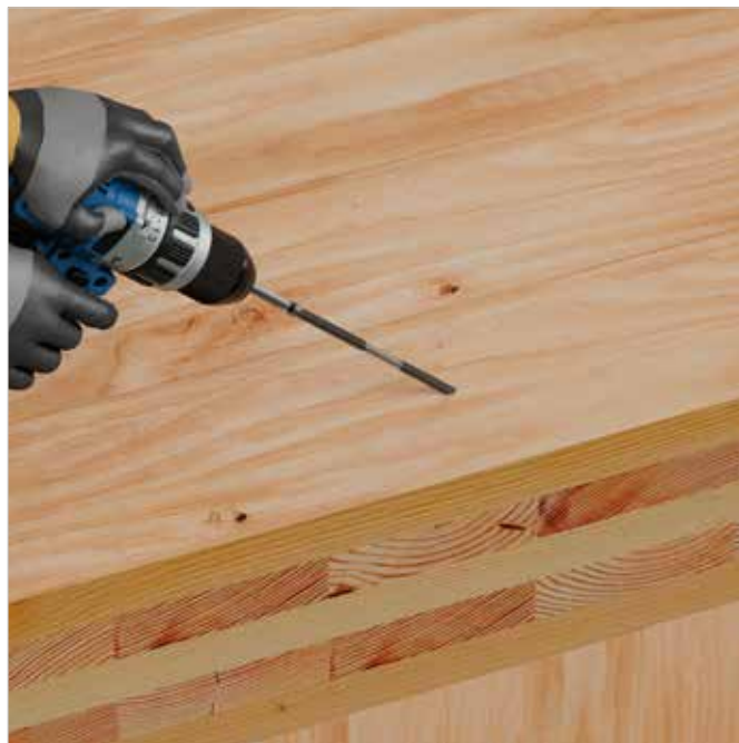
SWD screws in a CLT floor-to-wall application.
