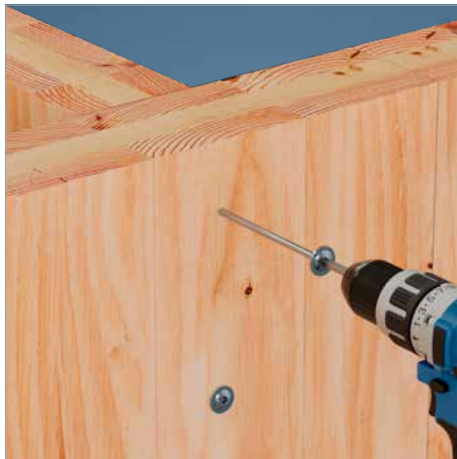
SWW screws in a 90° T-connection between two CLT walls.
